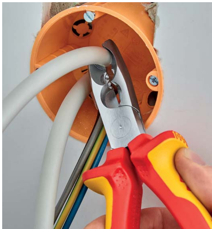
Stripping cable inside deeply mounted flush sockets
